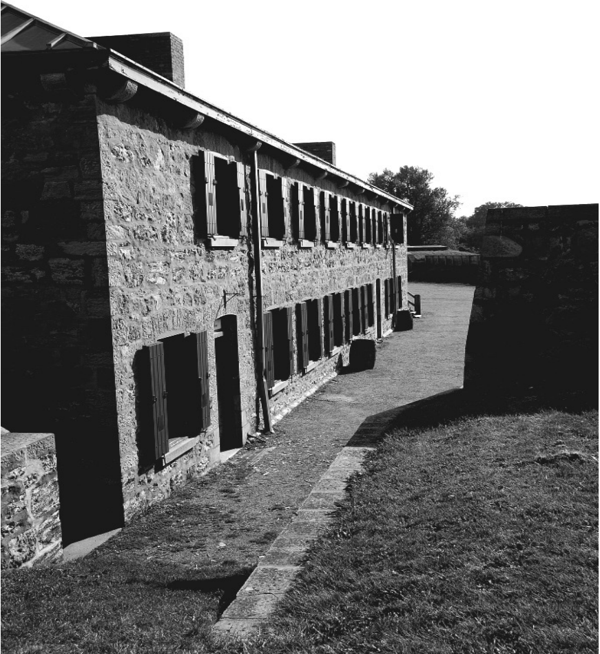
Figure 38. View from the Northeast Bastion toward the Stone Building.
